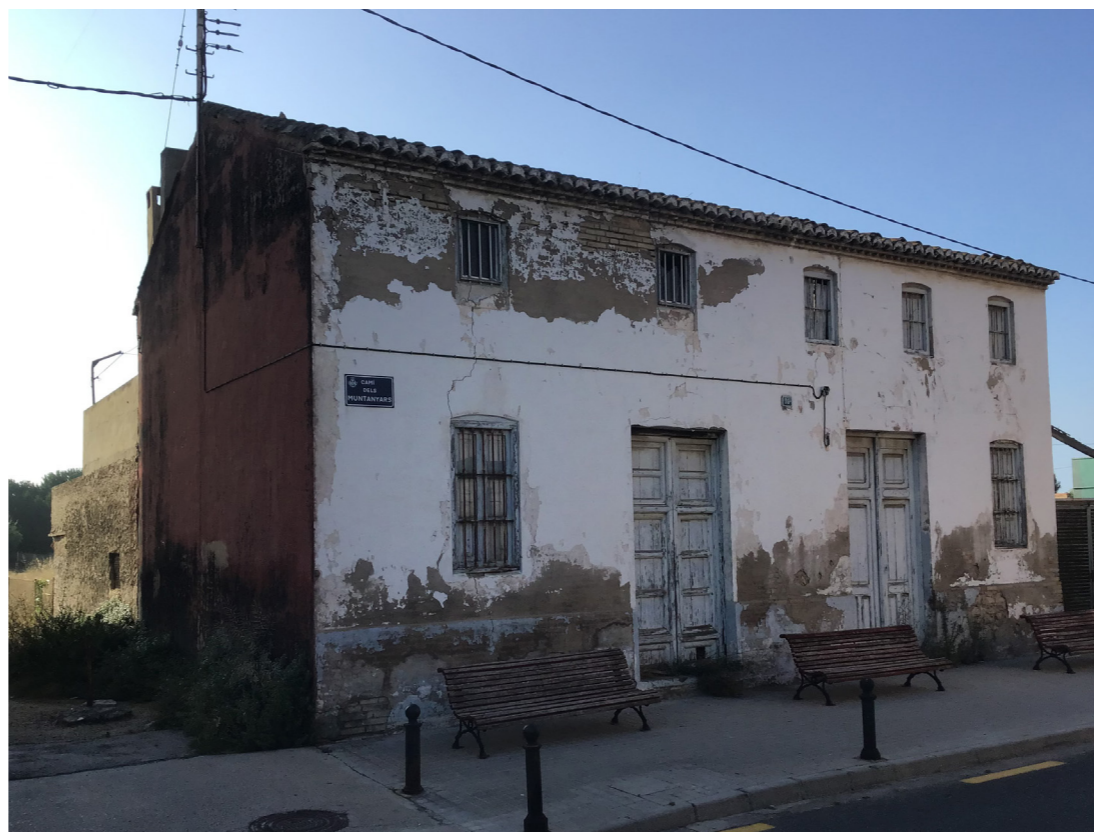
Building that is located on the plot of the project
