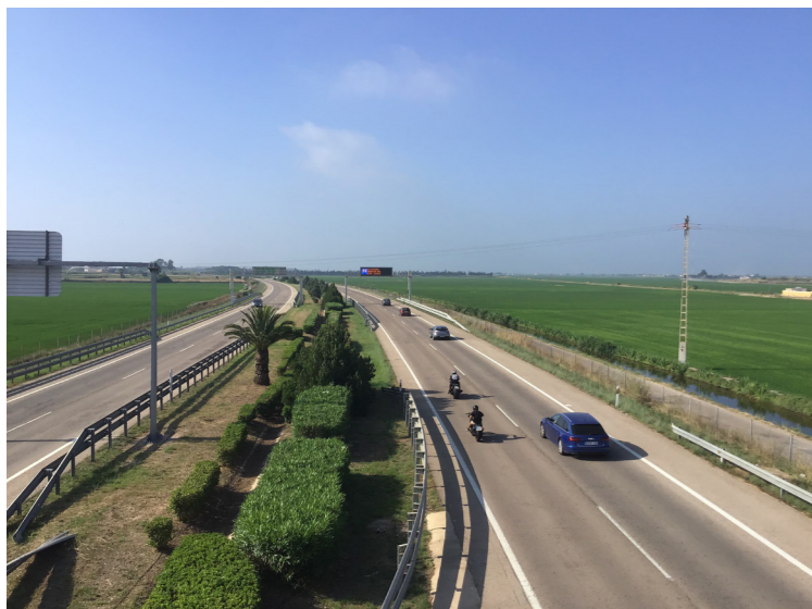
Views towards Albufera from the footbridge
