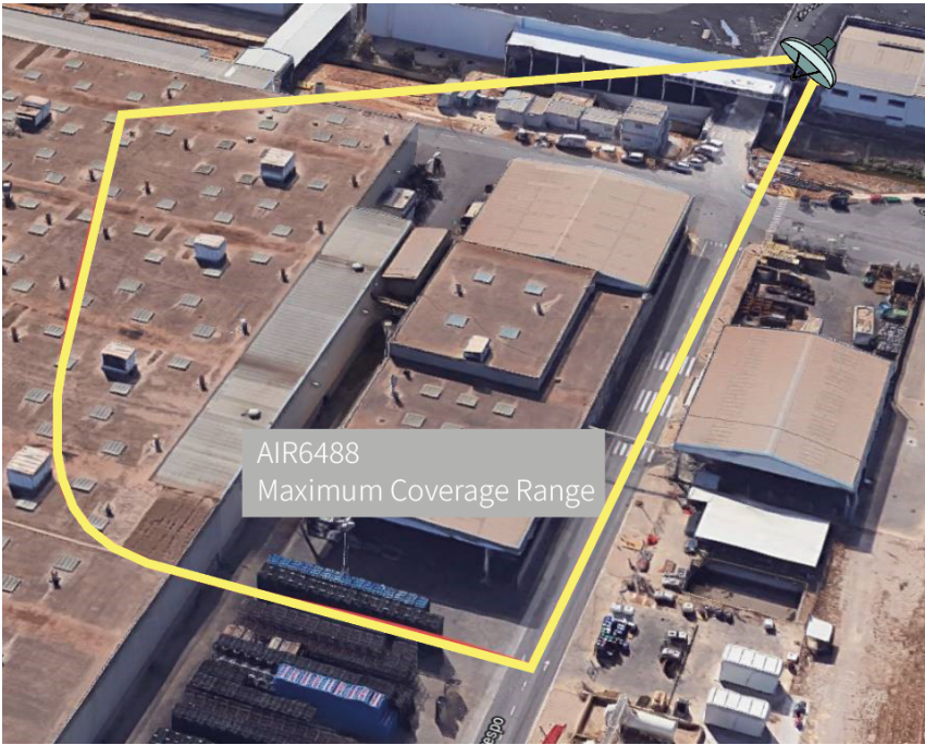
Figure 22: Outdoor antenna AIR6488 coverage.
