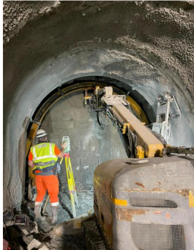
Figure 20: Pose du cintre
