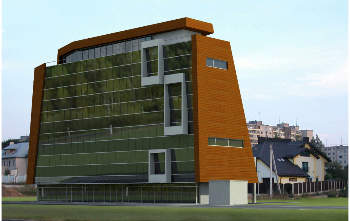
IMAGE 2 AND IMAGE 3. Final view of the construction.
