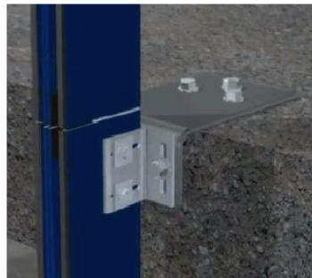
3 VERTICAL STEEL PROFILE INSTALATION
