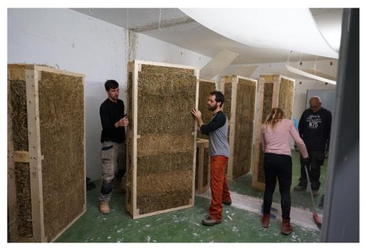
Figure A3. Moving the panels
