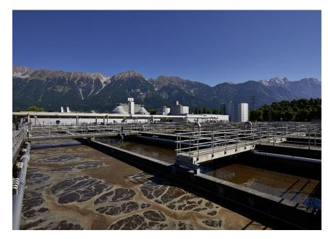
Figure 6 - Sedimentation tank in a purification plant (https://www.bmlrt.gv.at/fotoservice/wasser/ abwasserwirtschaft/IKB\_6205\_bah.html, with kind permission of the BMLRT, Austria).
