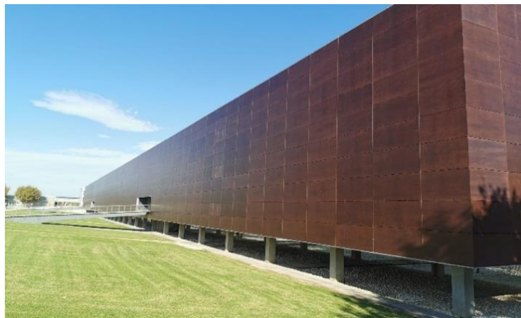
Figure 16: Building 8 west facade
