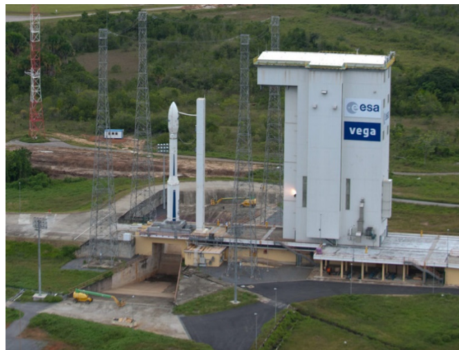
Figure 1: VEGA's launch pad. The channels for exhaust gases are observed below the rocket.
