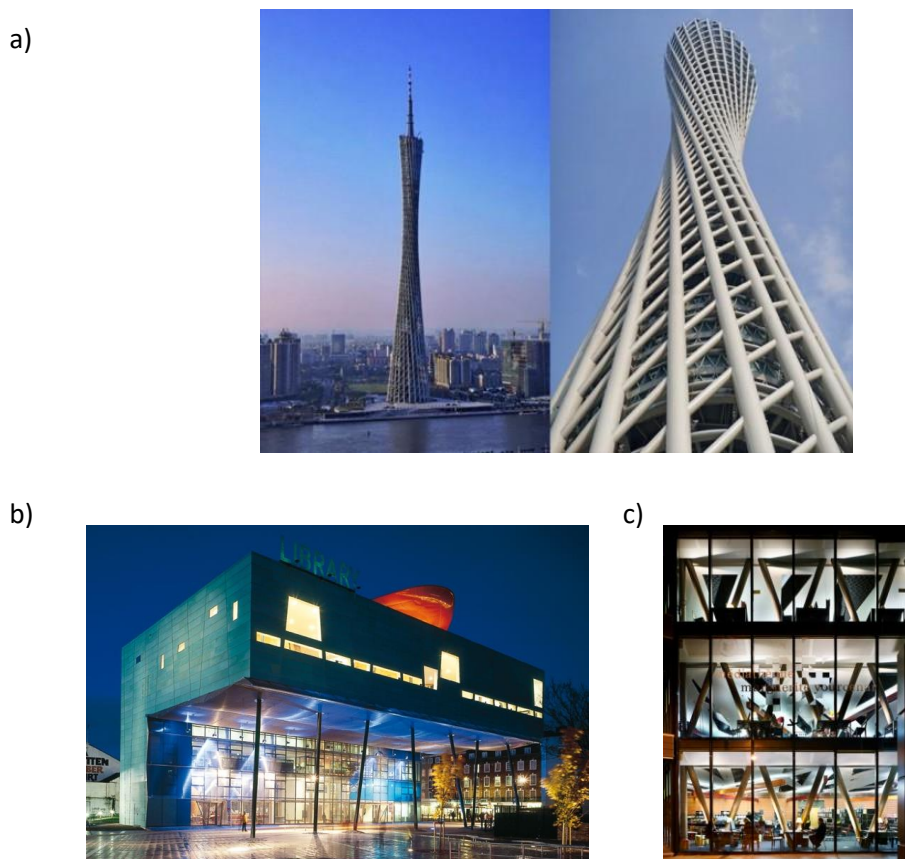
Figure 2: Examples of buildings using CFST columns: a) Canton Tower (Guangzhou, China); b) Peckham library (London, UK); c) Marguerite Yourcenar Media Library (Paris, France) [6]
