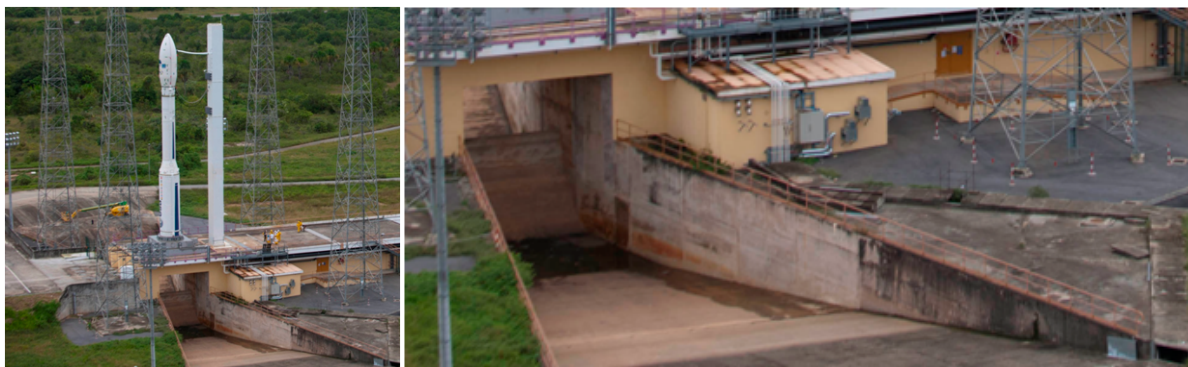
Figure 1: Pictures of VEGA launch pad: (left) general view and (right) detail of one of the ducts.
