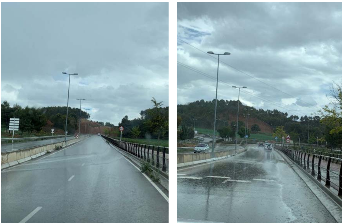
Figure 15. Flow across the road likely to cause hydroplaning (author: Beatriz Aranda).
