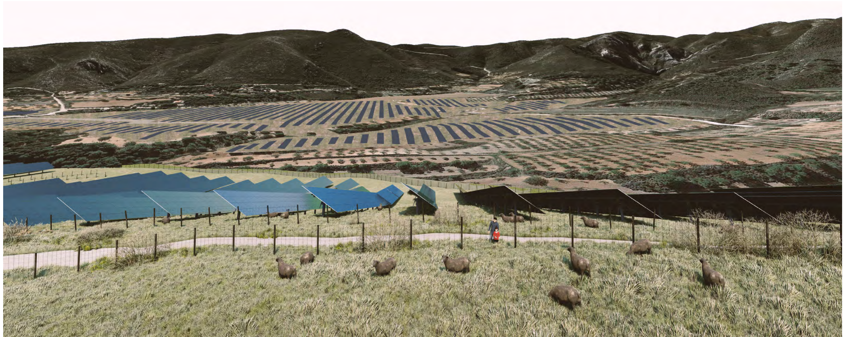
A combination of AutoCAD, Civil3d, Sketchup, Google Earth Pro, and Photoshop were used to determine the approximate location of the proposed solar arrays. The terrain in the foreground was modeled and rendered, then later combined with imagery from Google Earth Pro to produce the background image that depicts the extent of panel placement in the landscape. The installation of the solar modules actually opens up the viewshed of the surrounding mountain range.
