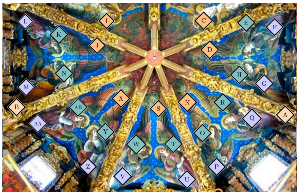
Figure 1. Approximate location of the probes and sensors at the apse vault of the cathedral of Valencia. Details of the installation of the probes and a scheme depicting the installation of probes in the frescoes can be seen in [1] and [2]. The image shows the position of the 29 probes for monitoring the relative humidity (RH) of the indoor atmosphere, displayed in different colors according to their position. Seven probes were located on the ribs (orange), two at the cornice (light orange), ten on the walls below the severies (purple), and ten probes on the frescoes (green).
