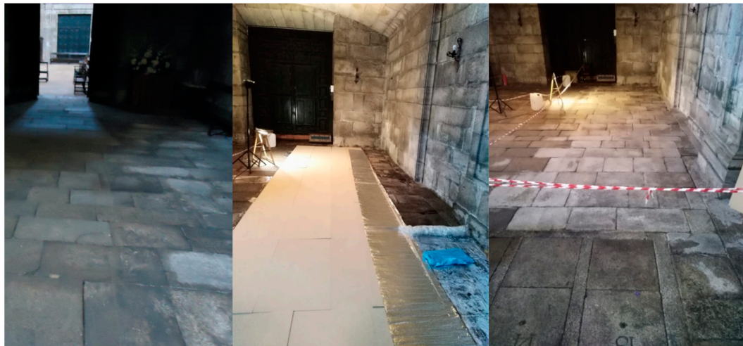
Figure 4. Detail of a church granite pavement 25 m 2 treated area following the high dimension bio-desalination optimized protocol. Area before treatment (left image), area during treatment (middle image), and area after treatment (right image).
