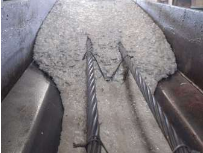
Fig.4. 2 Concrete pouring into the formwork
