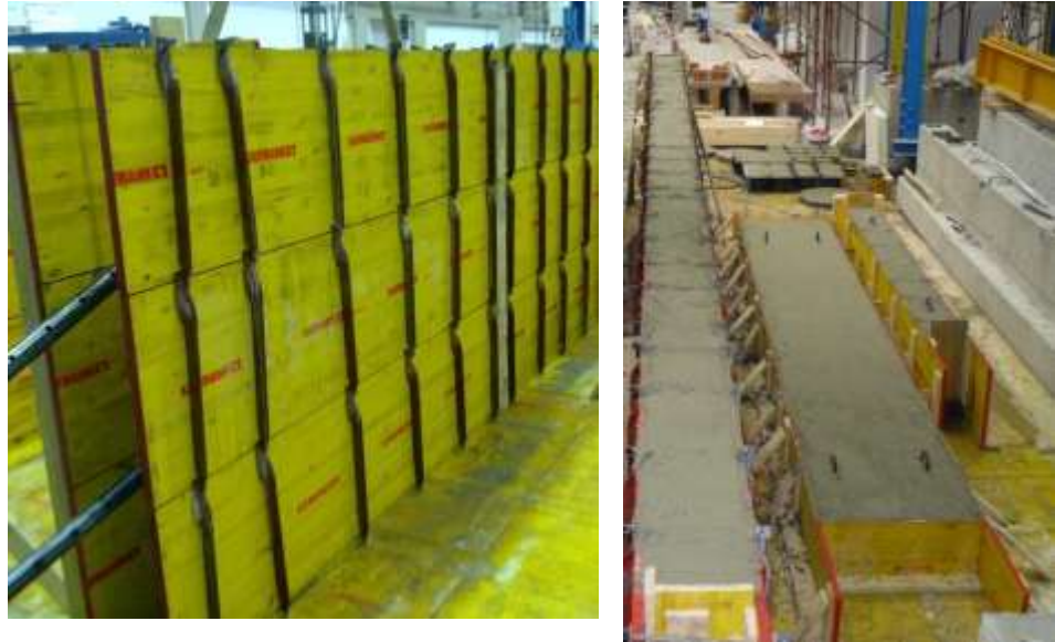
Fig.5. 11 Formworks and beams just casted
