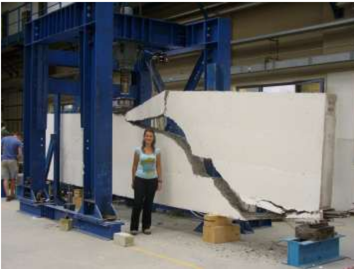
Fig.5.15 Beam H1500-FRC75 after its failure
