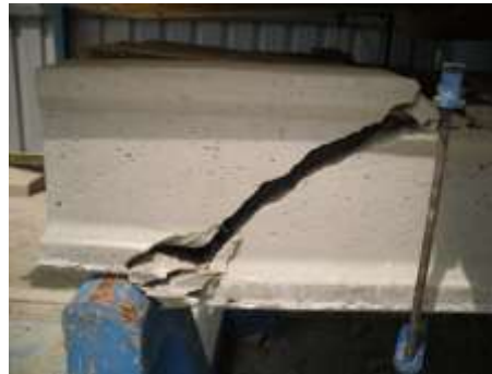
Fig.7. 10 Crack caused by tension shear and anchorage failure simultaneously
