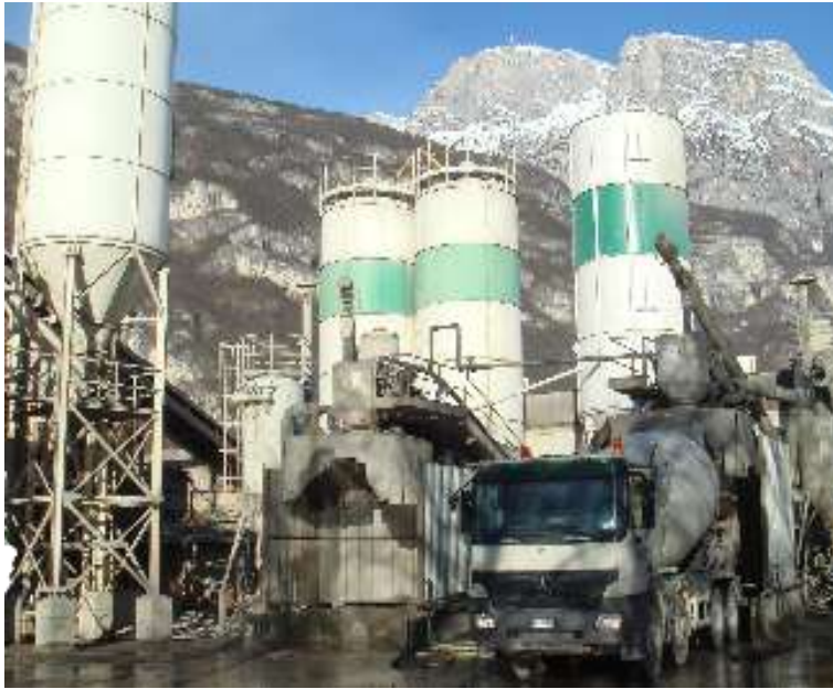
Fig.5.1 Concrete manufacturing plant
