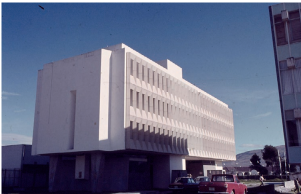
Fig. 4. Building of the Faculty of Mechanical Engineering, Escuela Politécnica Nacional. Oswaldo de la Torre, 1963 (Source: Oswaldo de la Torre's personal archive 2016).
