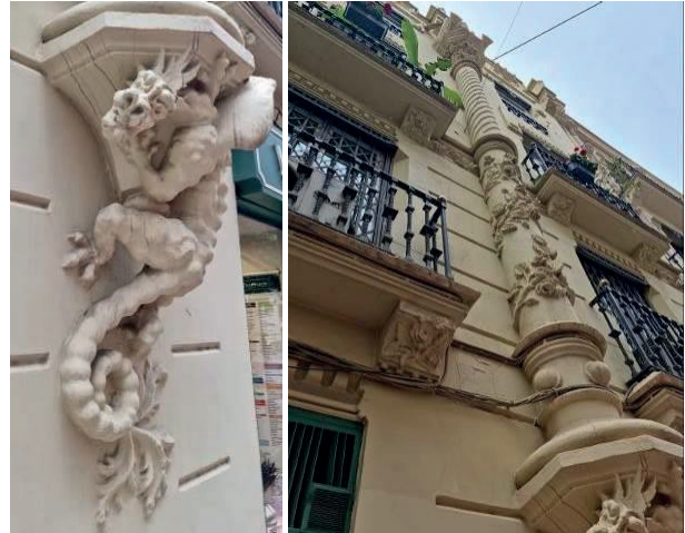
Fig. 14. Details of the decoration. The House of the Dragons. Cortina Building. At, 29, Cirilo Amorós street. Valencia (Source: The author).
