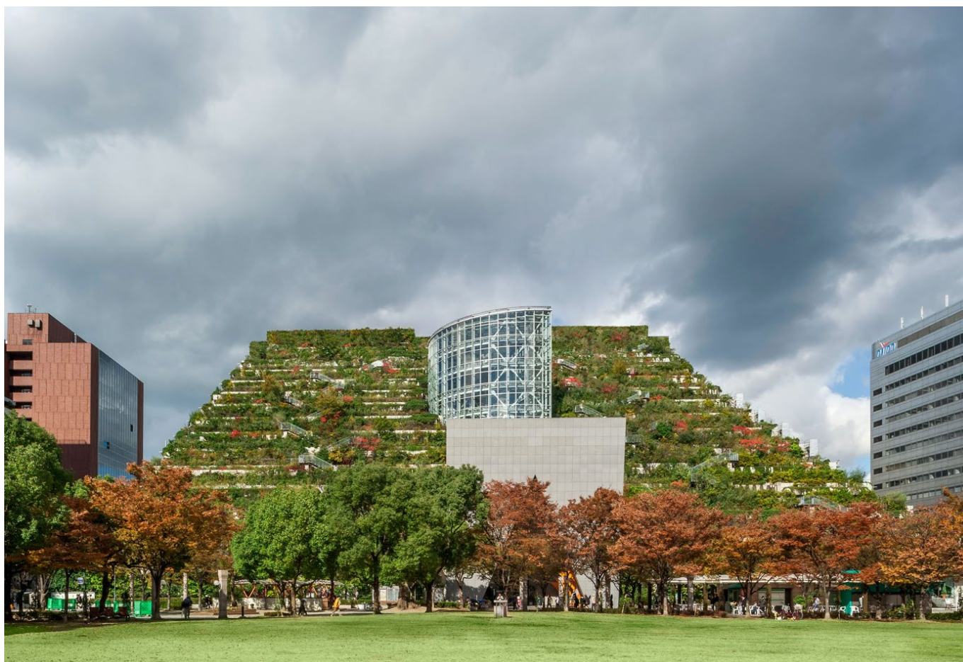
(Fig.17) Fukuoka Prefectural Hall. Recuperado de: https://www.greenroofs.com/projects/acros-fukuoka-prefectural-international-hall/
