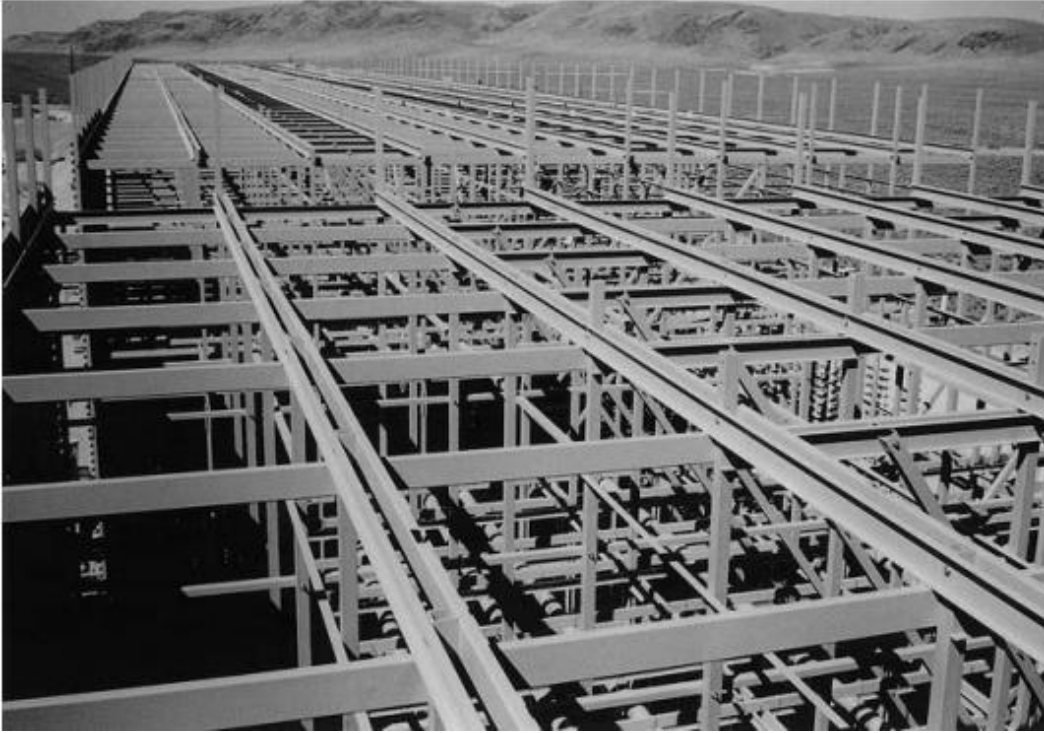
Figure 17 Water cooling tower structure (Courtesy, Bedford Reinforced)
