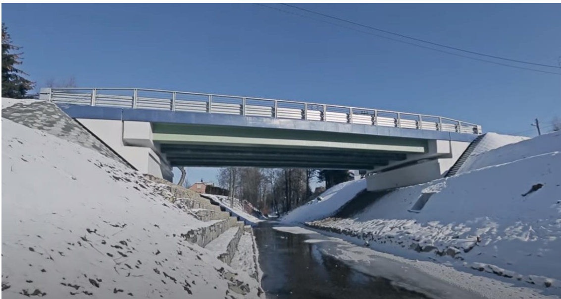
Figure 10 Construction of a bridge made of FRP composites
