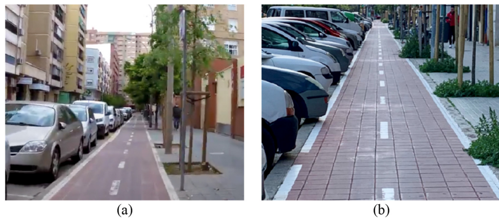
Figure 6. Sidepath without physical or vegetated curb next to parked motorized vehicles: (a) parallel parking, and (b) perpendicular parking.
