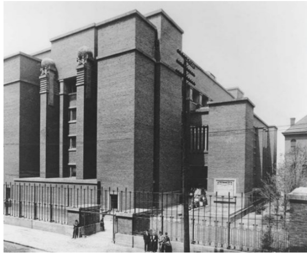
Figure 1.27. Frank Lloyd Wright, Larkin Company Administration Building, Buffalo, New York. Photo made in 1903. F.L. Wright Foundation, Taliesin West, Scottsdale, Arizona.
