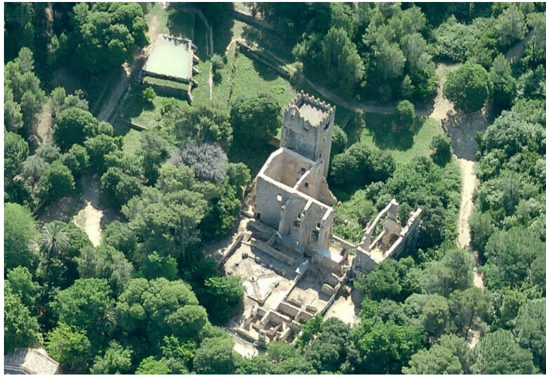
Fig. 1 - Aerial image of the current state of the remains of the monastery.
