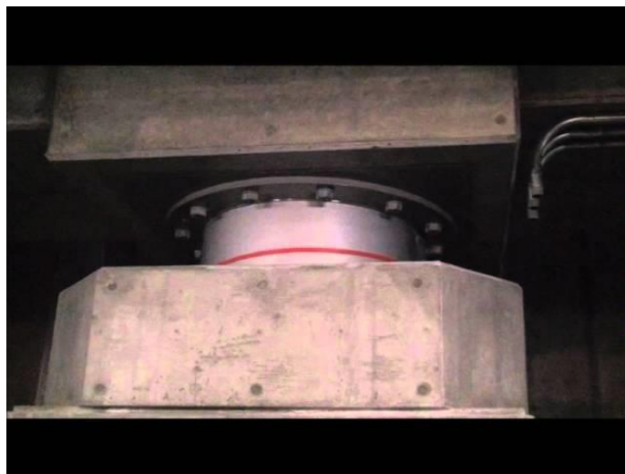
Photo 18 Measure against earthquakes
