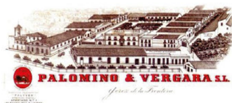
Fig. 3. Sherry building complex made by the basilica model reiteration (Source: Saldaña Trigo & Repeto Prieto, 2009, p. 130)
