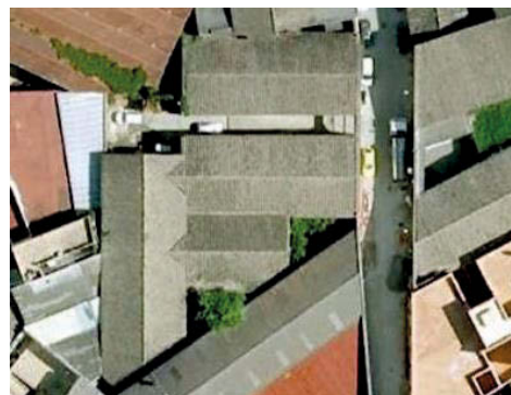
Fig. 7. Small complex articulated by the marginal spaces generated by the formal autonomy of the basilica cellars (Source: Google Earth, 2008).
