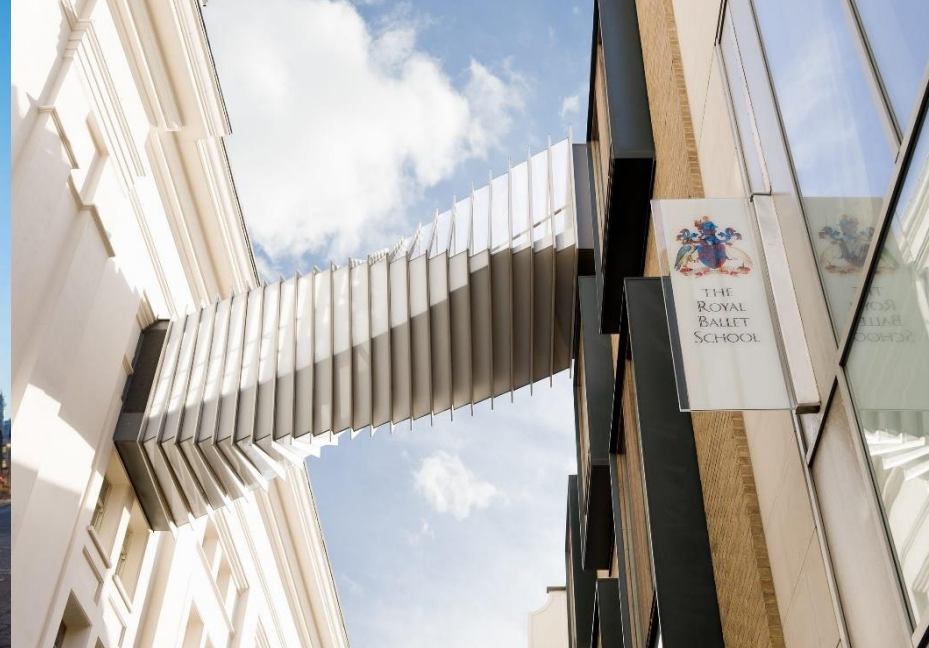
Figura II.197. Retorcida pasarela que conecta con la Royal Ballet School, Wilkinson Eyre
