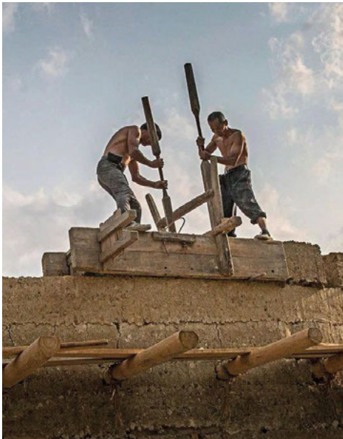
Fig.12 The formwork used in Tulous (Source: Chen, 2016, www.163.com/dy/article/E9GLU3K10521AJ1J.html )
