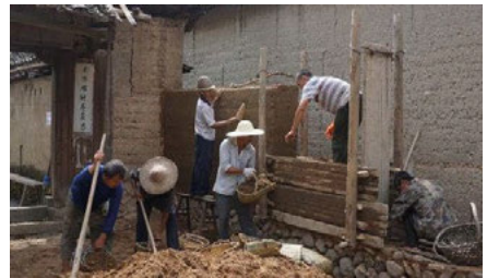
Fig.9 The formwork in southern Zhejiang (author,2019)
