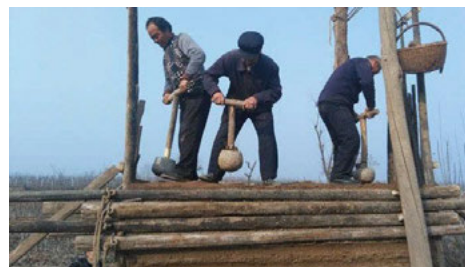
Fig.4. Rafter method used in Shanxi (Source: Zhang, 2017)
