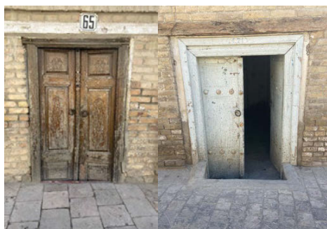
Fig. 4. Feature 4 of the traditional Bukharian Jewish houses: low narrow entrance door (IICAS, 2022)
