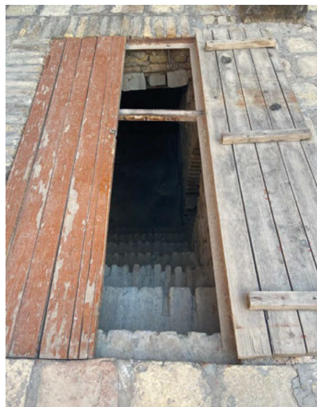
Fig. 6. Feature 6 of the traditional Bukharian Jewish houses: cellars system, a brick staircase connecting the cellars system and the lower courtyard with the upper courtyard (Source: IICAS, 2022)
