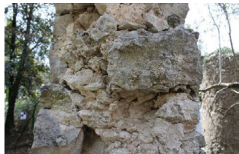
Fig. 11, 12. Details of castrum 's masonry (2021).
