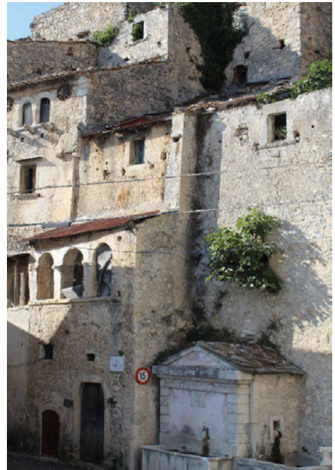
Fig. 4. Buildings of Pesche's historic centre (2021).
