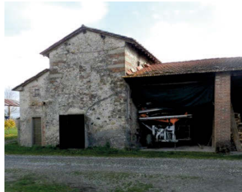
Fig. 7. Ancient drying room in Anghiari (AR) (Source: Manuela Mattone).
