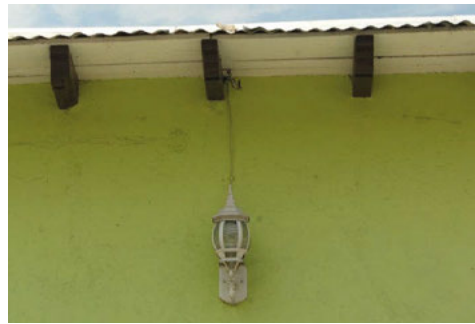
Fig. 1. Replacement of curved clay tile roof with galvanized sheets. (Parra Zebadúa., 2021)
