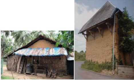
Fig. 4. Large overhangs built with local materials: [a] Goa – India (2019) [b] Normandy – France (Source: Patte, Architectures En Terre ).
