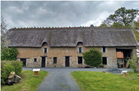
Fig. 5. Plants on roof ridge protected buildings from water damage, Maison des Marais in Normandy – France (2015).
