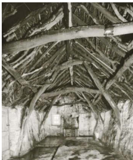
Fig. 3. Cruck framed roofs ensured the stability of roofs, Dumfriesshire – Scotland (Source: Walker, McGregor, Conservation of Vernacular Buildings).
