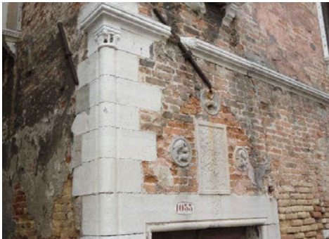
Fig. 3. Venice, Calle de le oche: detail of the gothic brickwork and a later cocciopesto plaster that have been bearing the effects of moisture and rising damp for centuries (Source: Squassina, 2012)
