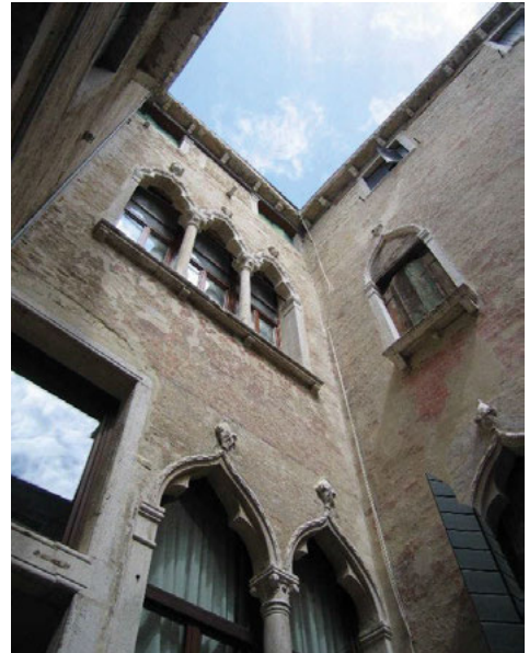
Fig. 1. Venice, Palazzo Moro: view of the inner court. The architectural features are emphasized by the medieval regalzier (false brickwork plaster), which is still well preserved (Source: Squassina, 2007)
