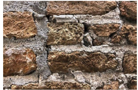
Fig. 4. Detail of medieval brickwork with well-polished lime-and-sand repointed joints (on the right) and a modern addition with a Portland cement mortar joint (left) highlighting the loss of traditional building skills (Source: Squassina, 2021)
