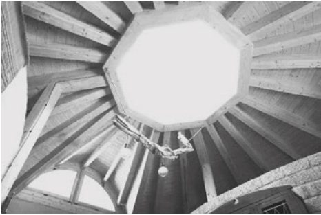
Fig. 7. Skylight, north-window and visible clay bricks
