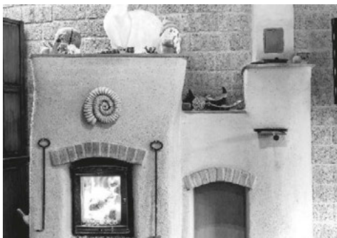
Fig. 12. Kachelofen built out of Bricks
