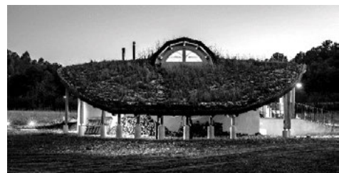
Fig. 9. Green Roof from the North
