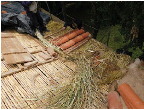
Fig. 8. Eaves with plant fibre fabrics in Casa del Marqués © Authors
