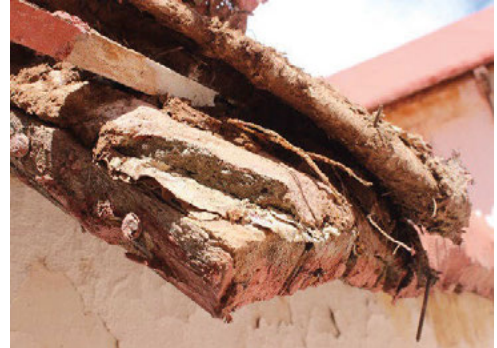
Fig. 6. Detail of the roof in Uquía © Authors
