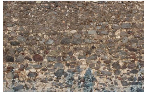
Fig. 3. Masonry of scheggioni in the masseria of Starza Regina (Source: Author 2021).
