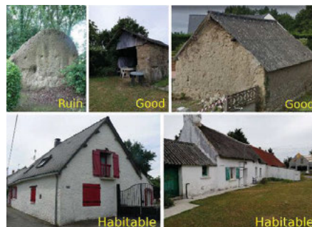
Fig. 7. Cob buildings in different states of preservation
