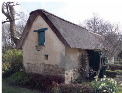
Fig. 1. A cob outhouse at Kerhebé, dating from the mid-19th century (Source: Hilton, 2015).
