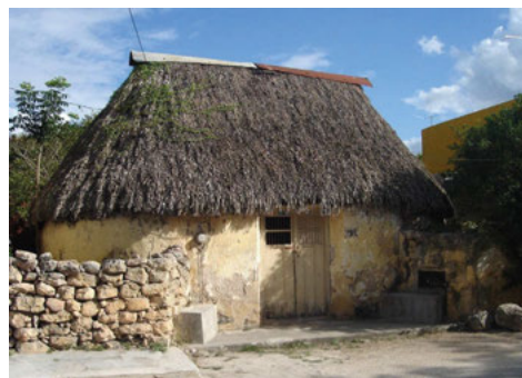
Fig. 1. Vernacular architecture of Yucatán “Mayan house” (Source: Guerrero, 2021)
