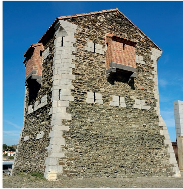
Figure 4. Vauban's freestanding towers. On the left, the Panissars tower associated with the Fort de Bellegarde; on the right, the Redoute Béar tower in Port-Vendres.
