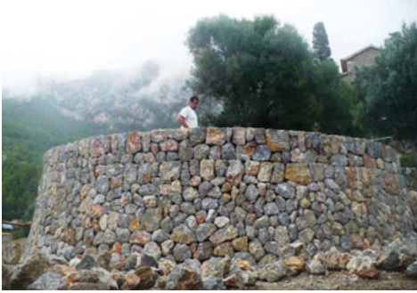
Fig. 4. Artífex Balear: Drywall course in Deià, s/f (Source: artifexbalear.org/con_tra )
