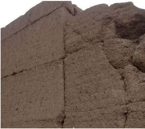
Fig. 7. Joint between modelled earth blocks. Huaca Tres Palos – Lima (Source: Torres, 2021).
