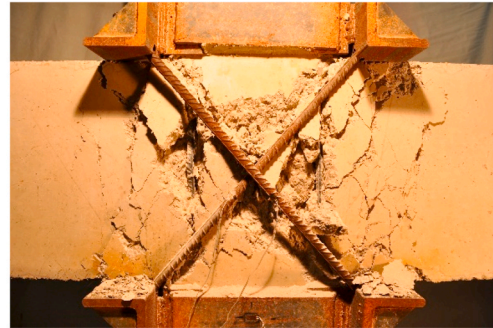
d. A.DB.L1-2 damage state after first cycle for the 3% drift ratio.
