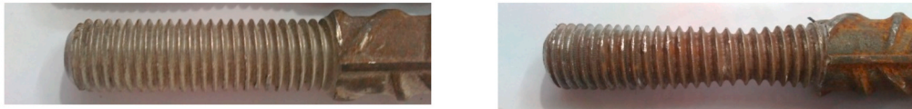
d. Plastic deformation with the reduction in the cross-sectional area on one diagonal bar
