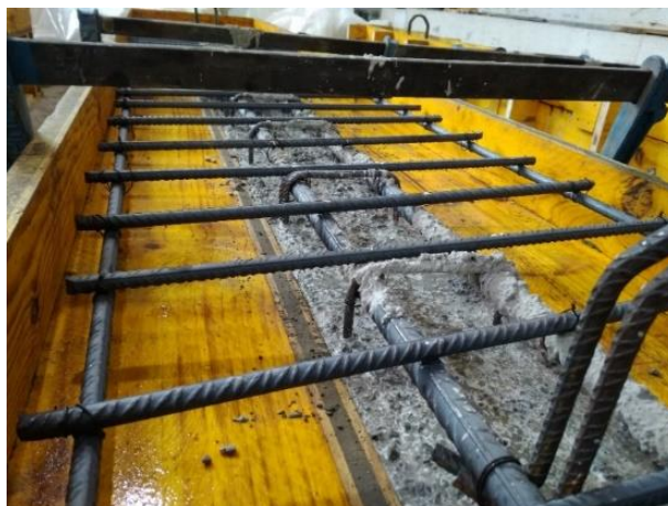
Fig. 4. “As cast” interface appearance before the cast-in-place slab’s concrete casting.
