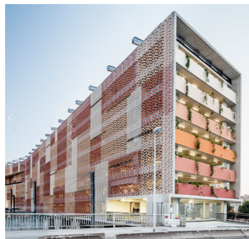
Archikubik Studio Parking Saint Roc, Montpellier CELOSÍA FACHADA
