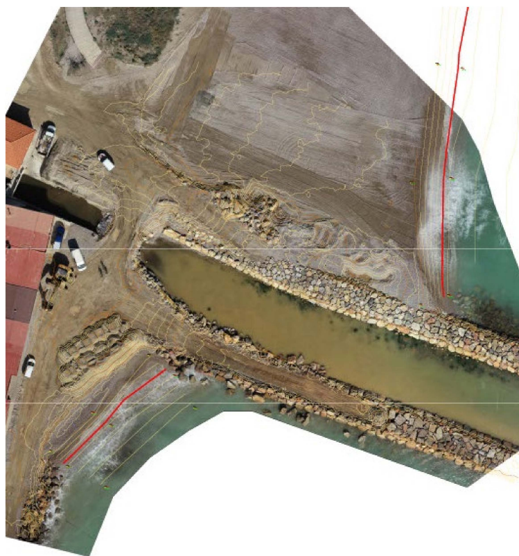
Figure 12. Orthophotography of defense coastal erosion works at Almenara and Sagunto beaches; ZL (red lines) and DTM (yellow lines) from UAV.
