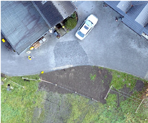
Figure 2. Aerial image detail view of a refurbished sinkhole. Image courtesy, RAG.
