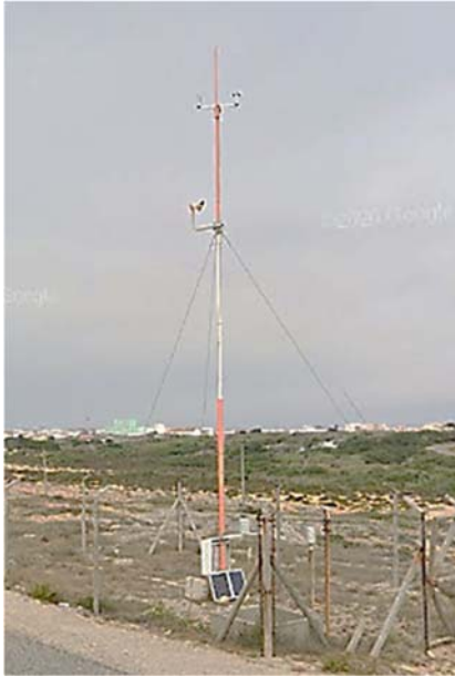
Figure 2. Peniche weather station.
