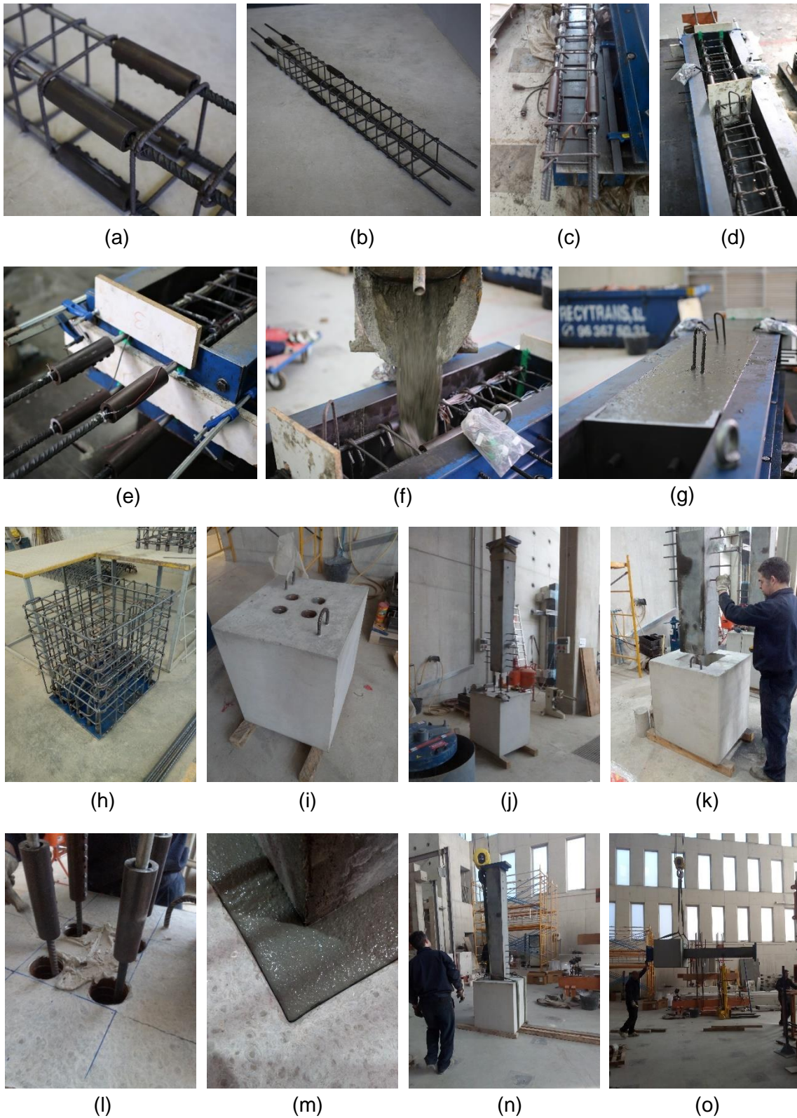
28 Figure 5: Manufacturing the specimens: (a) PB connection specimen reinforcement arrangement; (b) SP 29 connection specimen reinforcement arrangement; (c) NiTi SMA – steel coupler; (d) reinforcements into 30 formwork; (e) protruding bars sticking out of the formwork; (f) casting UHPC; (g) concrete casting concluded;
