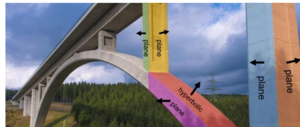
Figure 10. Segmentation of laser scanner data to define specific surface elements of a bridge (Wunderlich et al. , 2016).
