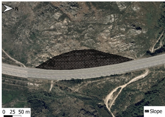
Figure 4. Slope adjacent to motorway.
