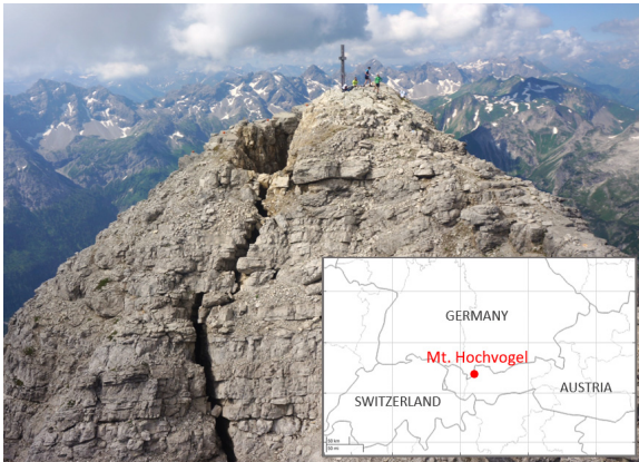
Figure 2. The summit of Mt. Hochvogel (2,592 m a.s.l.), located on the German-Austrian border, with its enormous cleft. The southern part (left part in the image) is moving several mm per month and threatens to break off completely.
