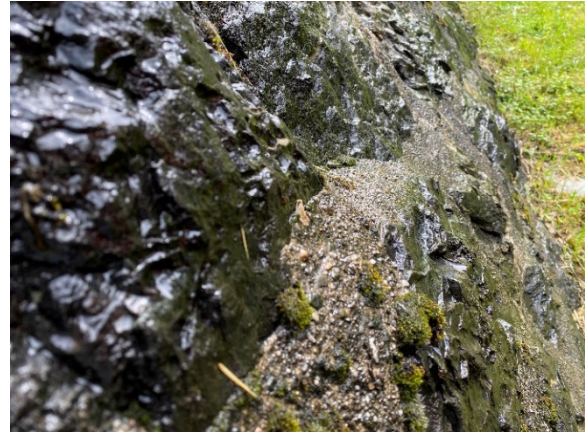
Figure 2. Challenging structure for geometric features as stone and joins have very similar surface characteristics and no clear topology.
