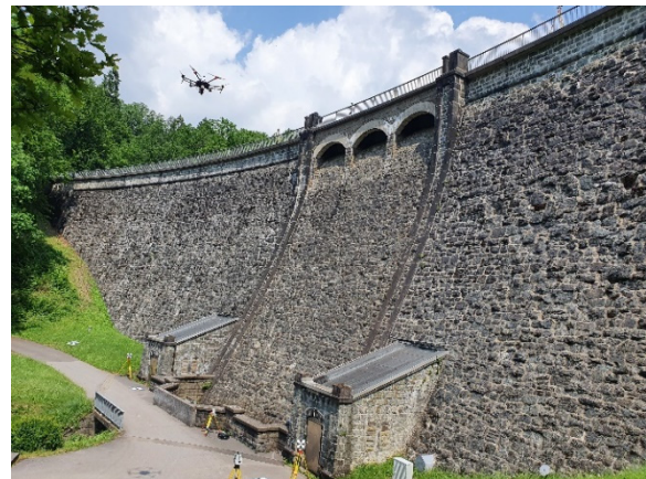
Figure 1. Water dam as monitoring object.
