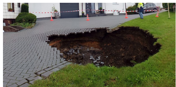
Figure 1. Near surface mining induced sinkhole. Image courtesy, RAG.
