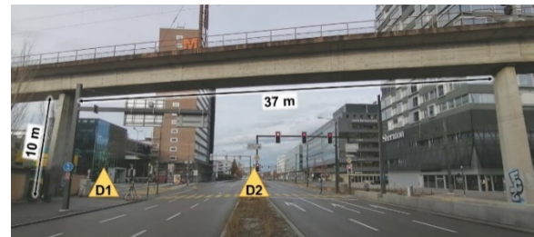
Figure 4. Investigated bridge segment and scanner positions at both measurement days (D1 and D2).
