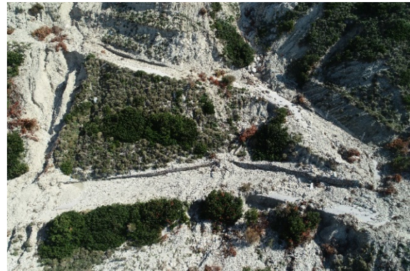
Figure 2. The infrastructure suffered extensive destructions caused by material relocation which resulted severe damage due to erosional phenomena and mudflows.
