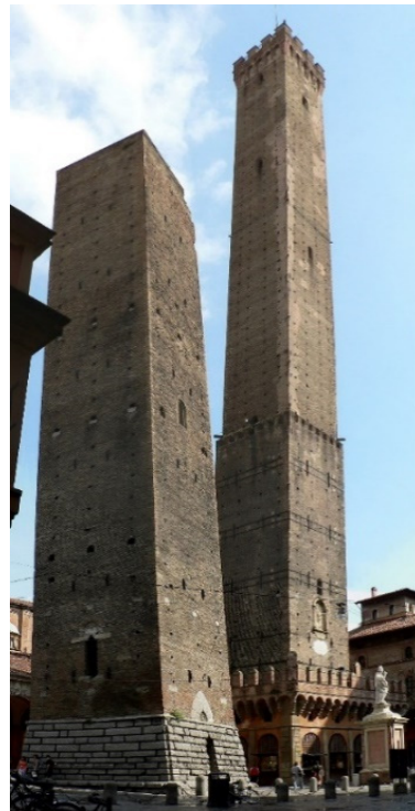
Figure 3. The two Towers: Garisenda (left) and Asinelli (right). The external side of the selenite basement of the Torre della Garisenda is clearly visible, as well as the entrance door.
