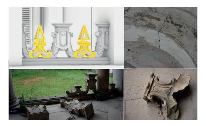
Figure 11 | Decorative elements and portions of architecture have been surveyed and catalogued. Through querying the three-dimensional model of the researched area, it is possible to have specific references to the observed object. These data converge in the database that constitutes the backbone of the 3D information system.
