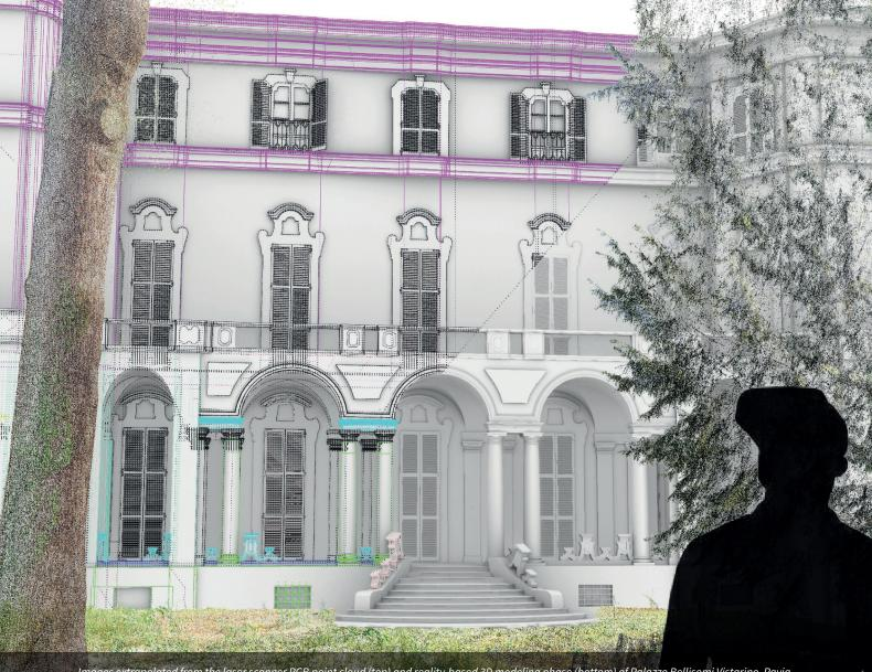
Images extrapolated from the laser scanner RGB point cloud (top) and reality-based 3D modeling phase (bottom) of Palazzo Bellisomi Vistarino, Pavia
