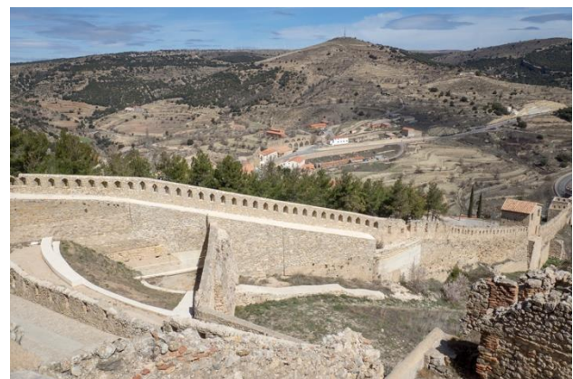
Figure 5. Section of the wall with a steep slope, between the Portal de la Nevera and the Castle (Source: S. Portela, 2018).
